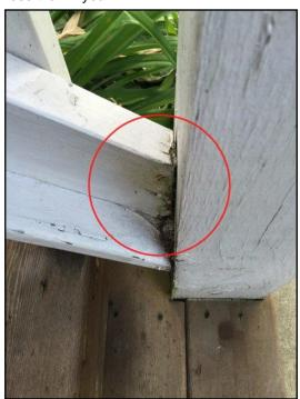
21. Condition: • Rot or insect damage The guardrail is rotted and extremely loose.
