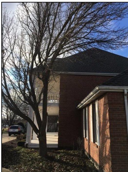
Trees or shrubs too close to building
