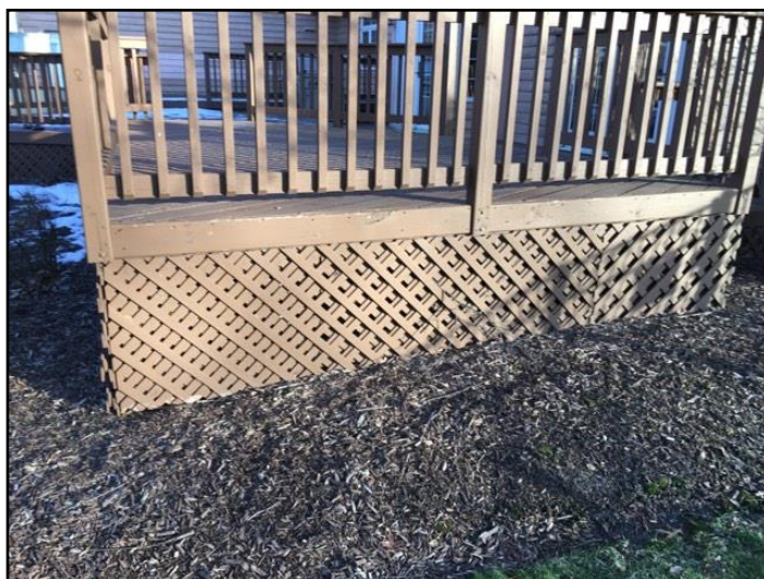
No Access Under The Deck
